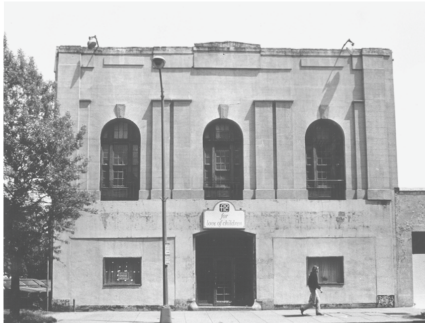
Constructed in 1904, the Belmont Garage was the first public automobile garage in Washington D.C. Its defining feature, large arched windows, has been preserved and restored at Liz.
